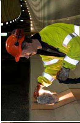
Tunnel cleaning is done both mechanically and manually.
