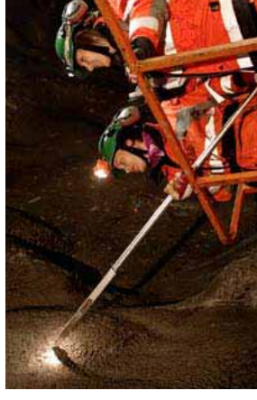
Inspection of the rock and rock reinforcement.
